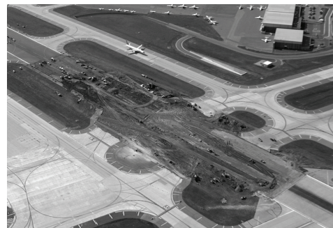
Aerial shot of runway construction - August 21 — Photo courtesy of Bordner Aerials
